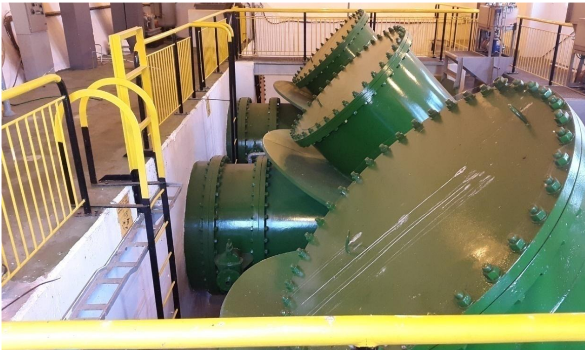
30) Outlet Tower: The three outlet pipes that supply water to the pump station
