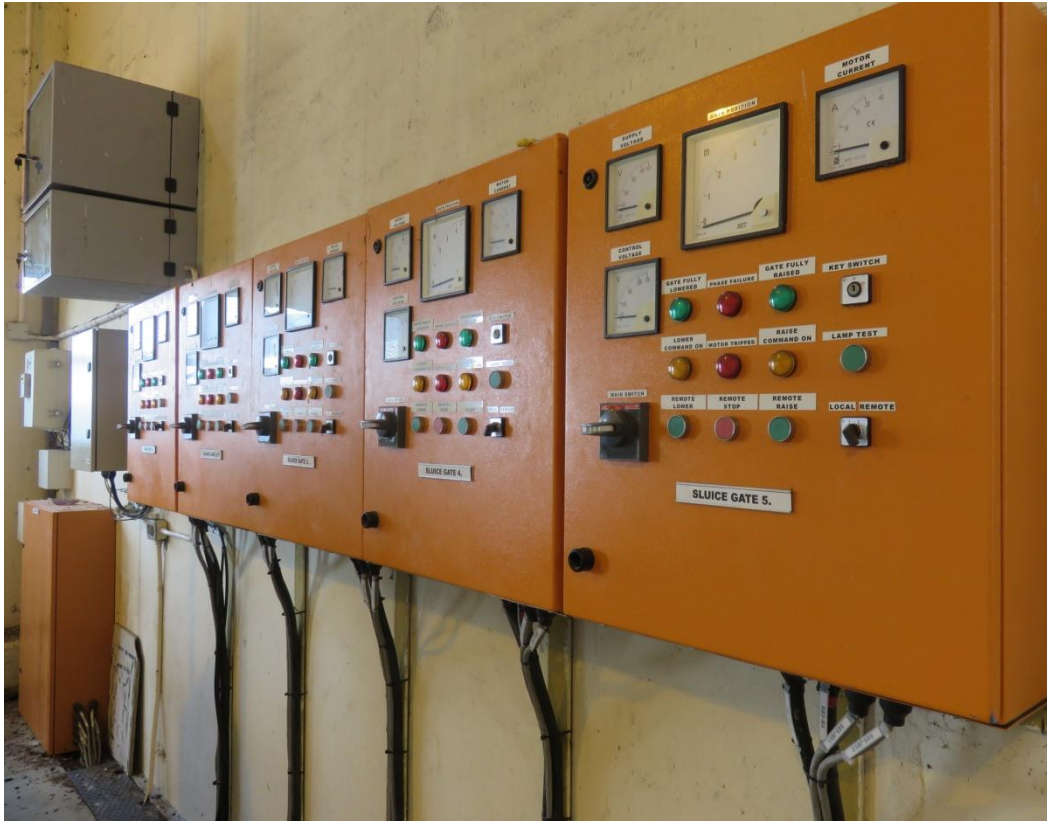
13) Control panels for the radial gates
