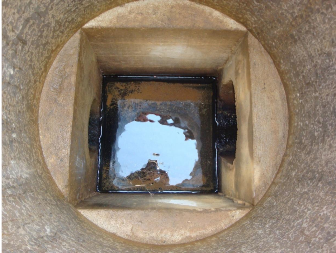
9) Slow flowing water in one of the tow drain wells close to the spillway
