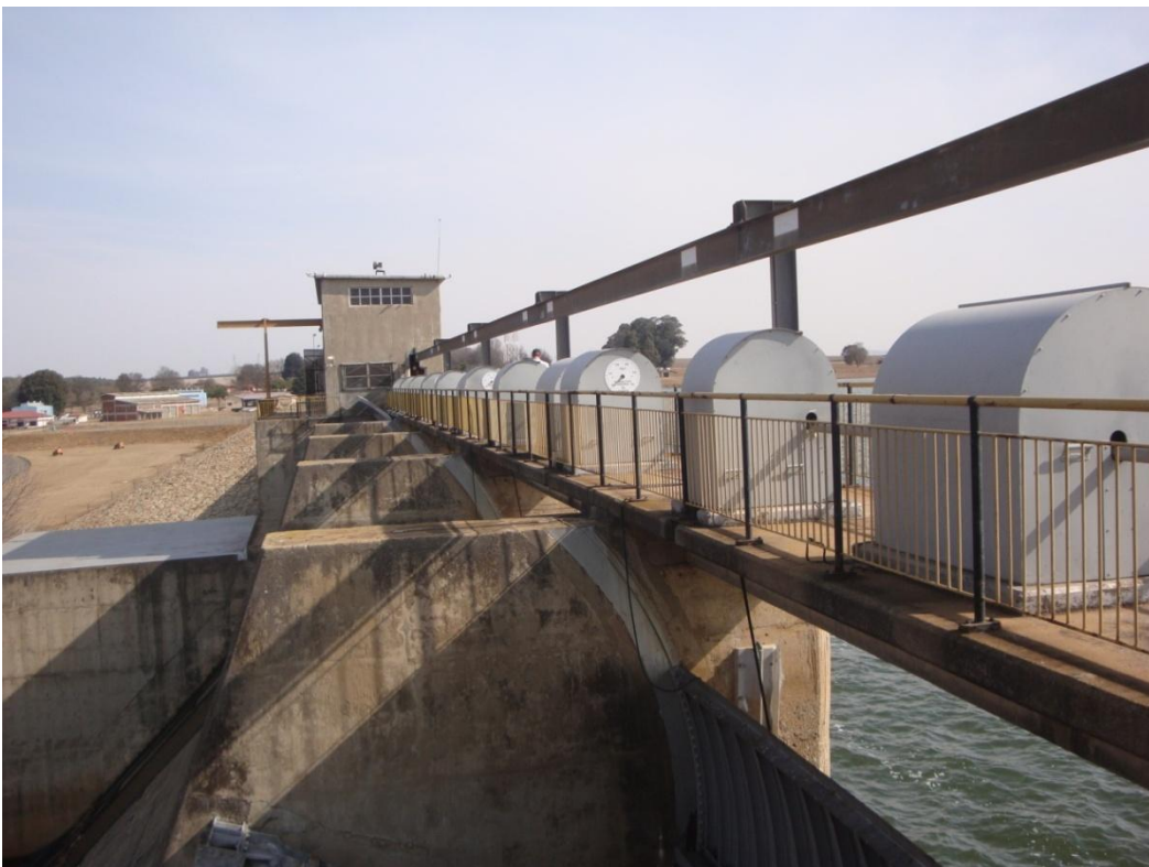
16) the spillway NOC with the radial gate control stations
